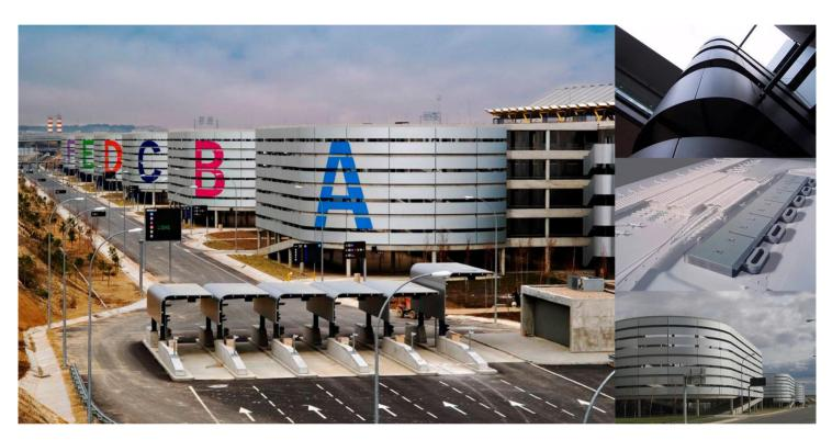
The car park building of the new terminal of Barajas Airport, of  $656,40 \times 80,00$  m on plan and six levels, is divided into six modules of  $112,00 \times 80,00$  m, without joints. Structurally, it is a 0,38 m deep reinforced concrete waffle slab, supported by a grid of columns of  $8,00 \times 8,00$  m.
